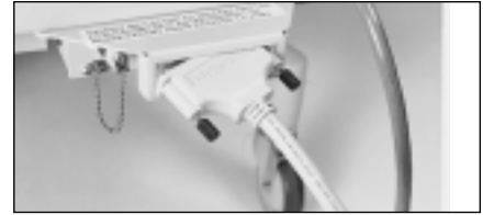
3. Communication Cable is unattached.
